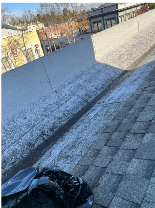
A view of the silt on the Mountain View 244 roof
